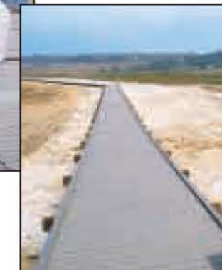
RIGHT: Completed section of the Boardwalk
