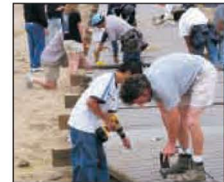
ABOVE: Boardwalk under construction
